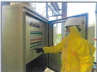
PO2 Stop NaOCl Pump at Panel
